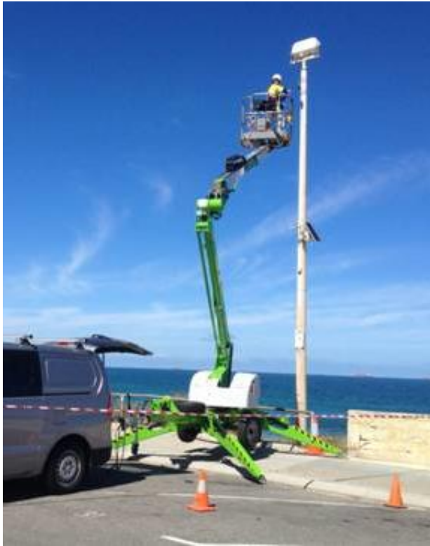
Figure 3.1 Remote imagery unit installation on the light pole in the main beach car park, opposite Overton Gardens
