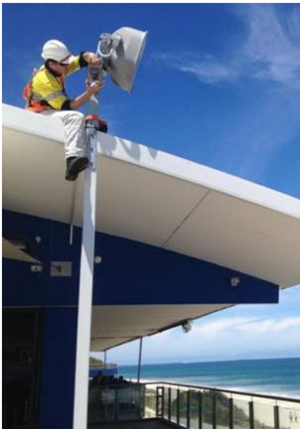
Figure 3.2 Remote imagery unit installation on the light pole on the North Cottesloe Surf Life Saving Club roof
