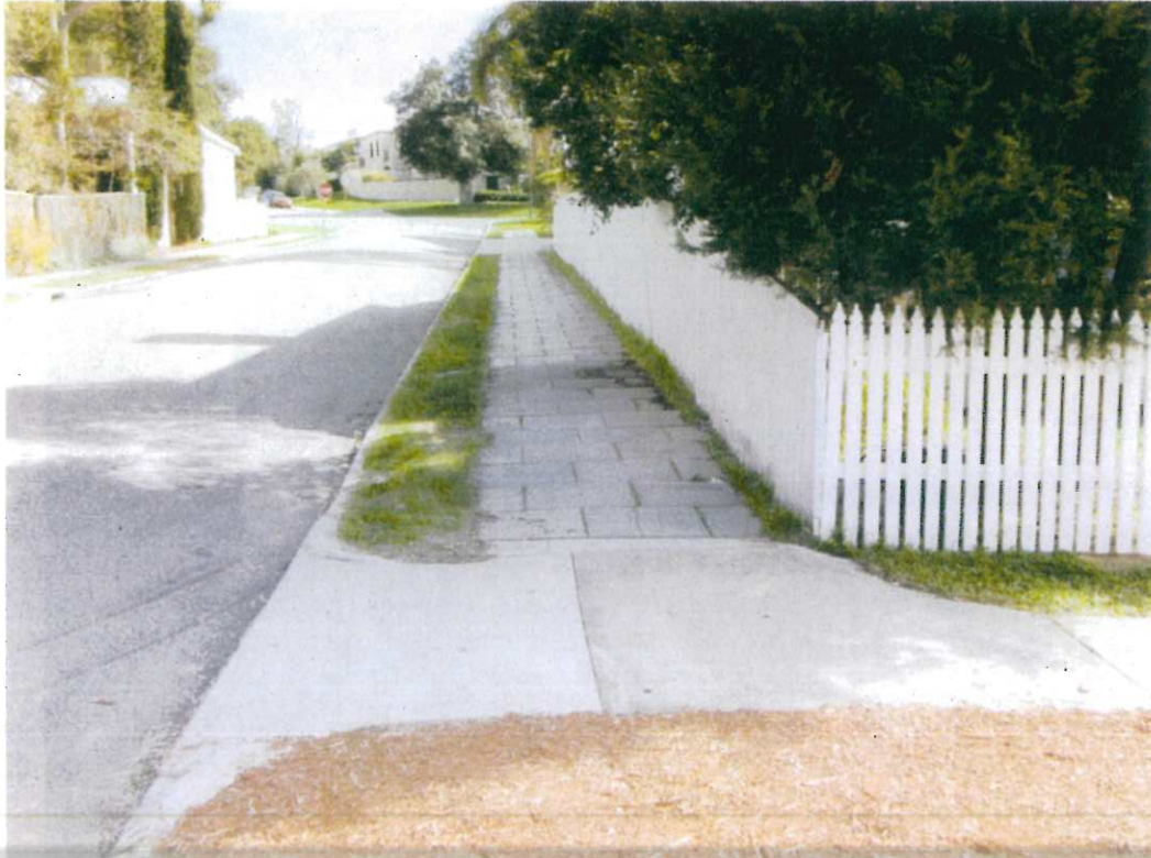
PHOTO 9 Princes St facing west Slab footpath may become a trip hazard
