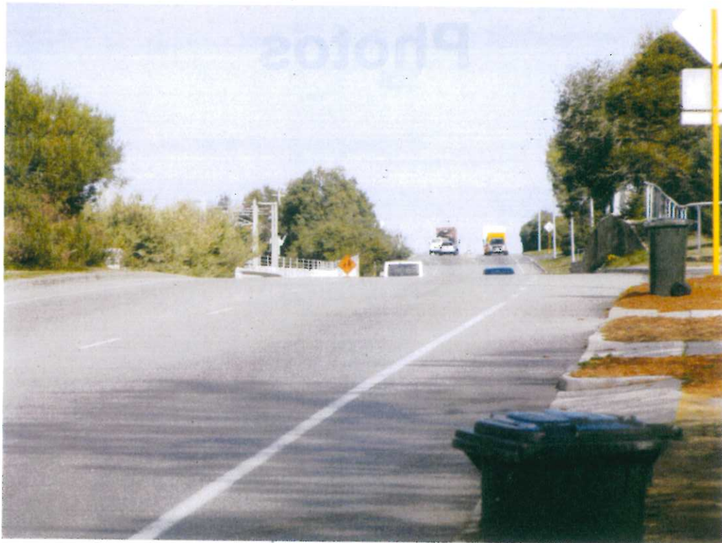
PHOTO 2 Curtin Ave just north of Princes St facing south Sight lines restricted by crest
