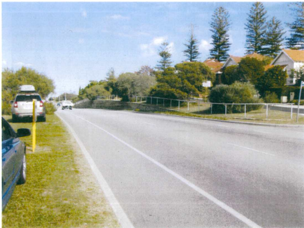
PHOTO 10 Curtin Ave facing south Bushes restrict sight lines,
