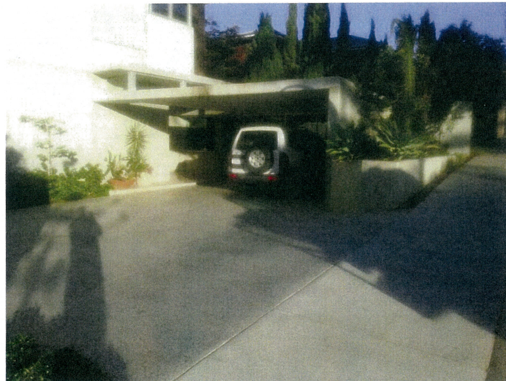
202 Broome Street - Flat Roof Garage, partly submerged by lie of the land, similar to our proposed 1.6m off the boundary
