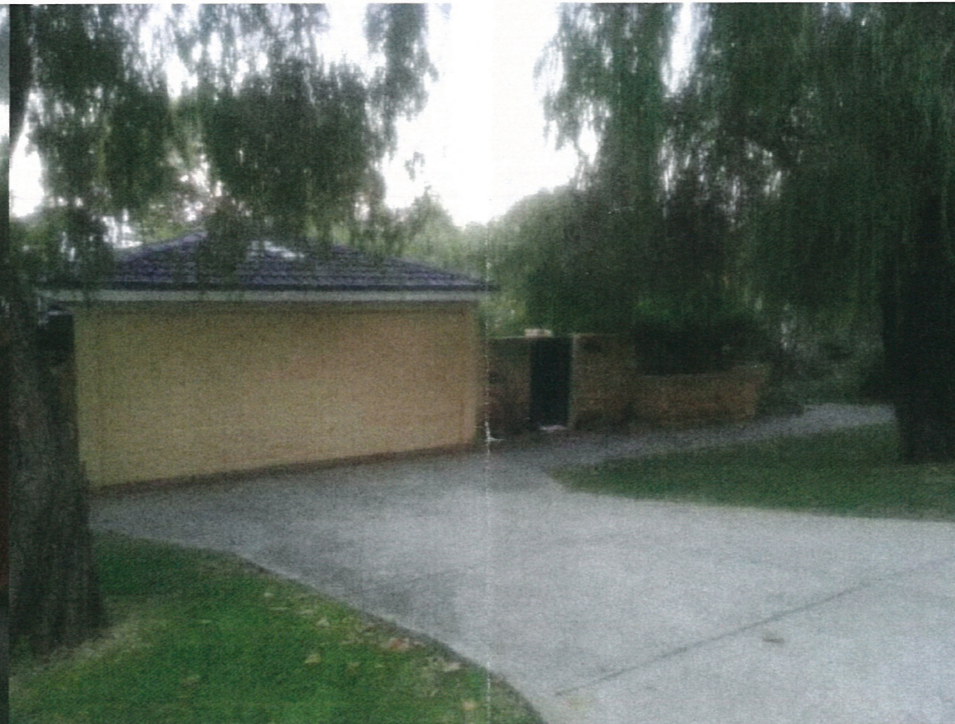
10 Deane Street 0.3m back from front boundary
