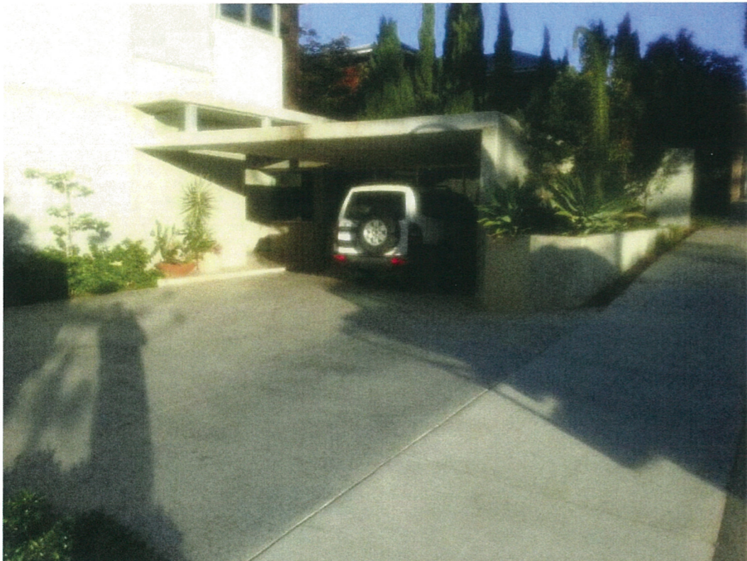
202 Broome Street - Flat Roof Garage, partly submerged by lie of the land, similar to our proposed 1.6m off the boundary
