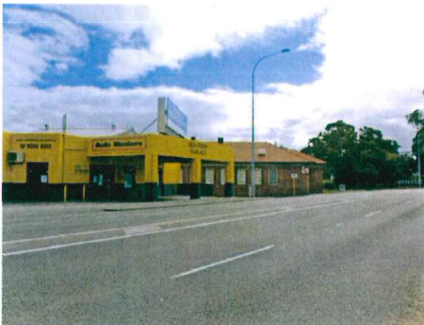
Telephone Exchange: view to northwest on Stirling Highway
