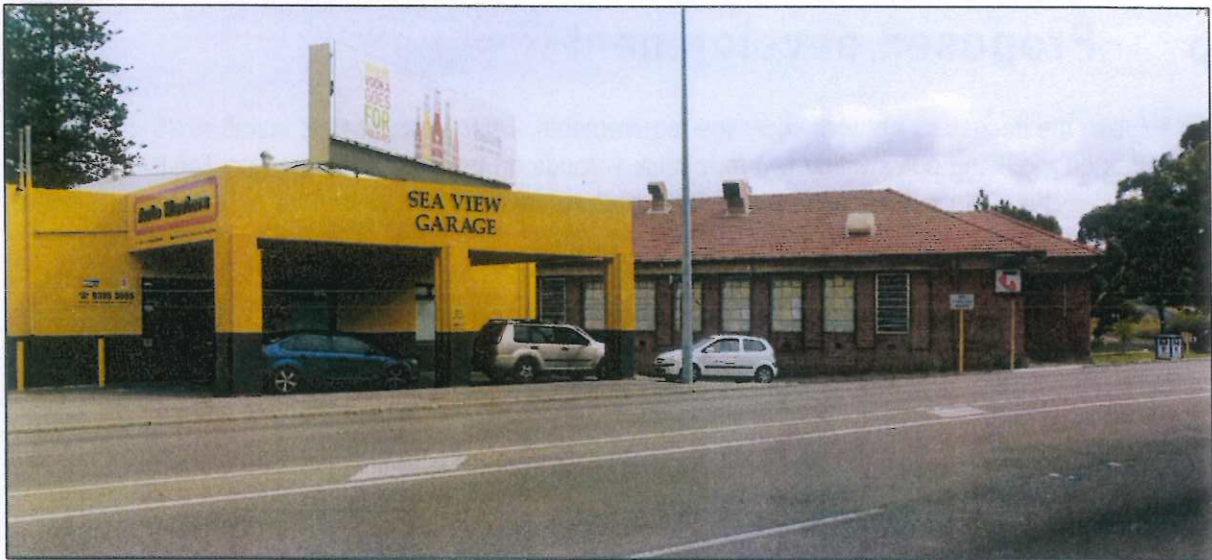
Photograph 1 – View of subject site looking north from Stirling Highway
