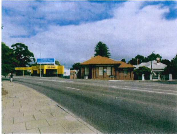
Telephone Exchange: view to west on Stirling Highway
