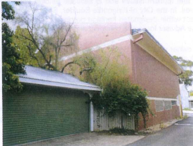
Telephone Exchange: Pennyfeather Lane and rear garage of No 3
