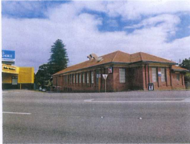
Telephone Exchange: corner view to northwest on Stirling Highway
