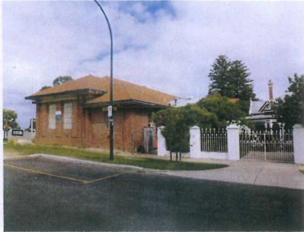
Telephone Exchange: Front view to southwest in Congdon Street
