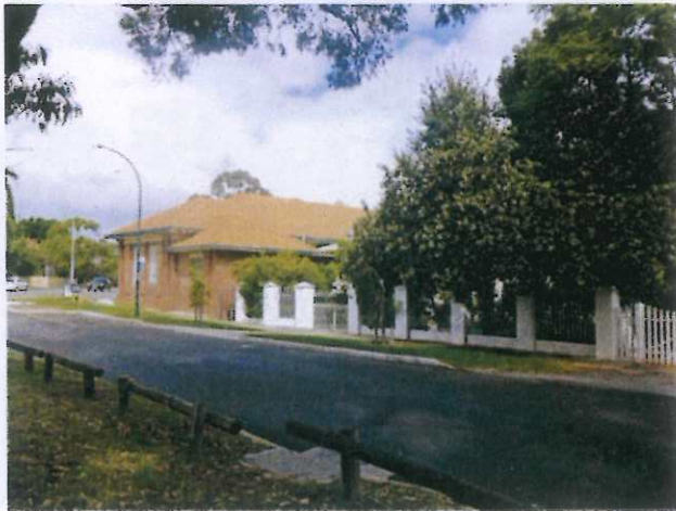
Telephone Exchange: View to south in Congdon Street (No 3 right)
