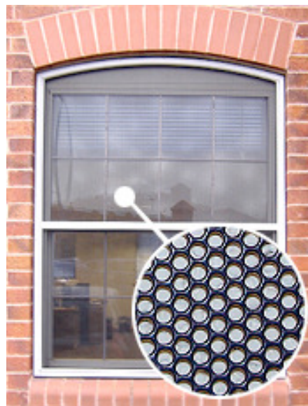
Use of toughened glass
