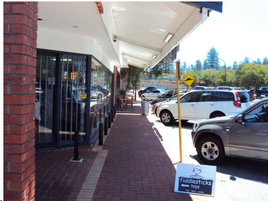
Existing bollards next to shop window
