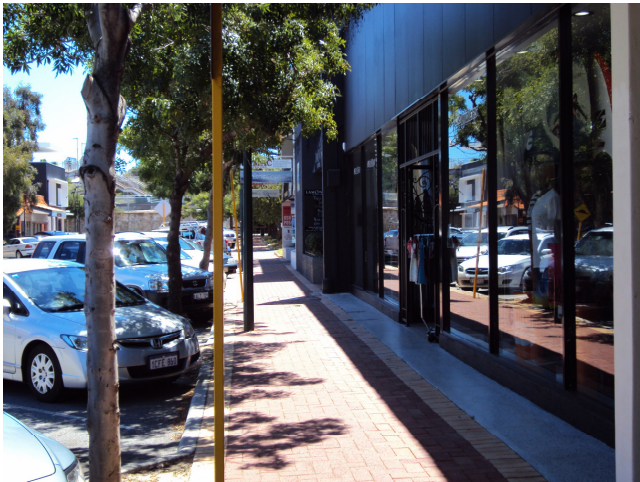
Mullions and internal grilles
