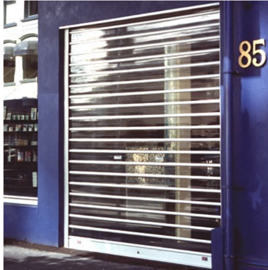
External grilles on shopfront
