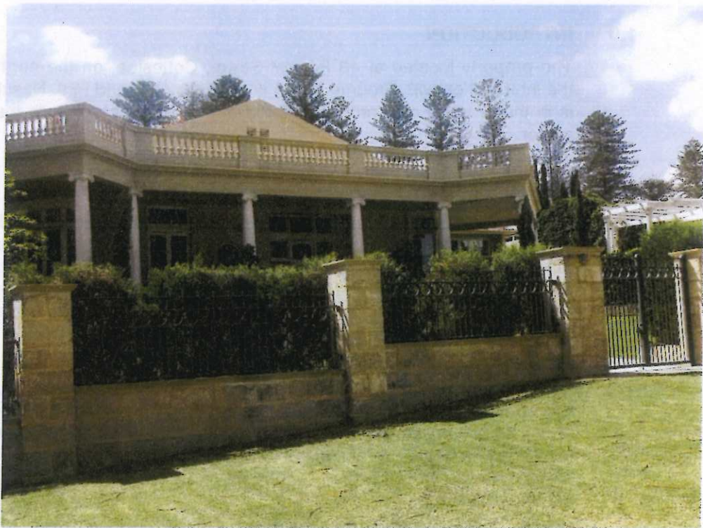
South elevation. September 2012.
