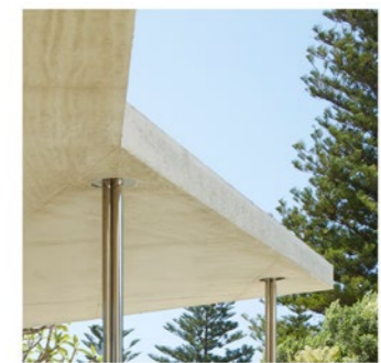
B Concrete canopy
