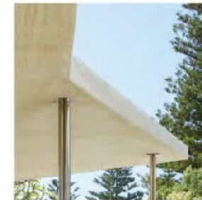
B Concrete canopy
