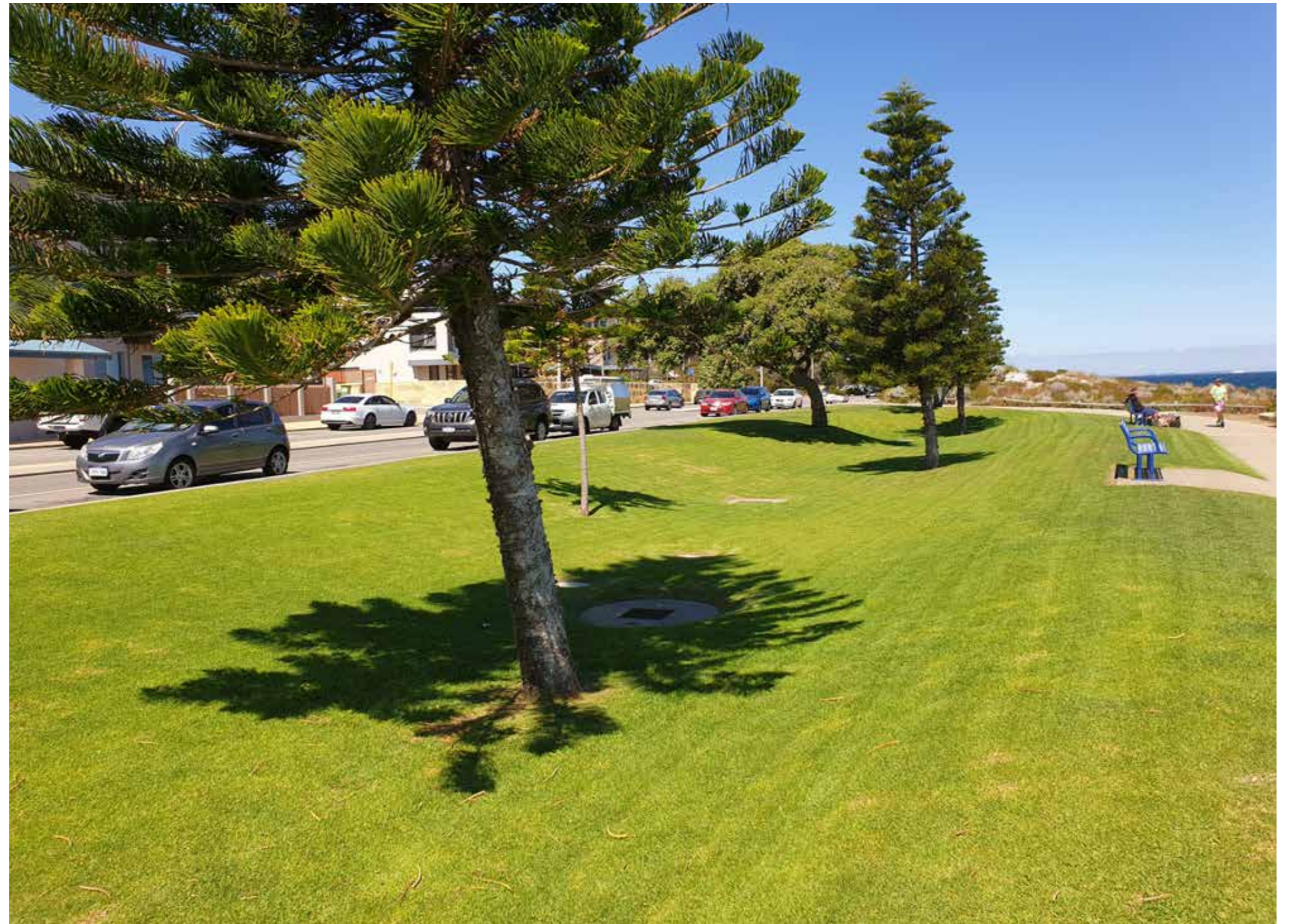
Image 7. Drainage Swale, udlia
