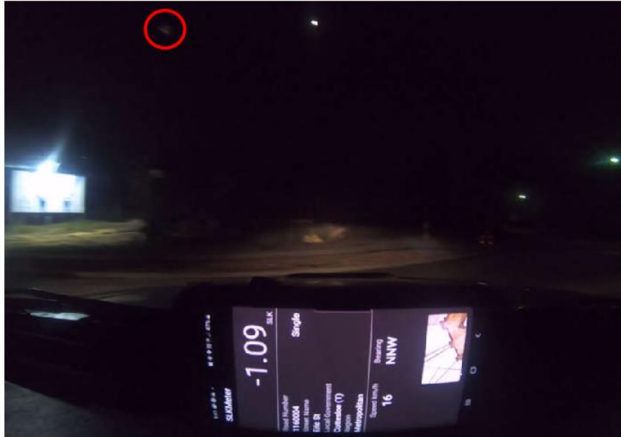
Photo 7: View from the roundabout northwards showing the poor delineation at the NW quadrant of the Eric St / Railway St roundabout due to the faulty street light (indicated in the red circle).
