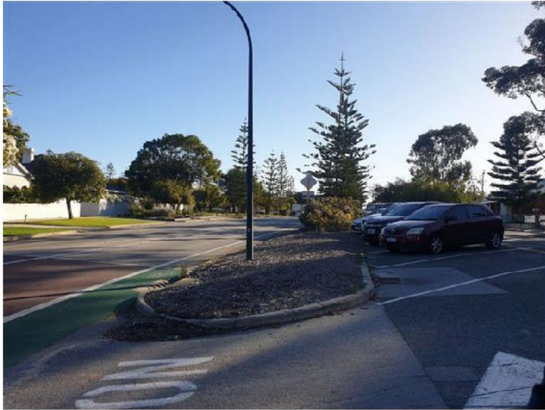
Photo 3: Sight distance to the west along Eric Street from the KissnRide exit is restricted by the Banksia trees.
