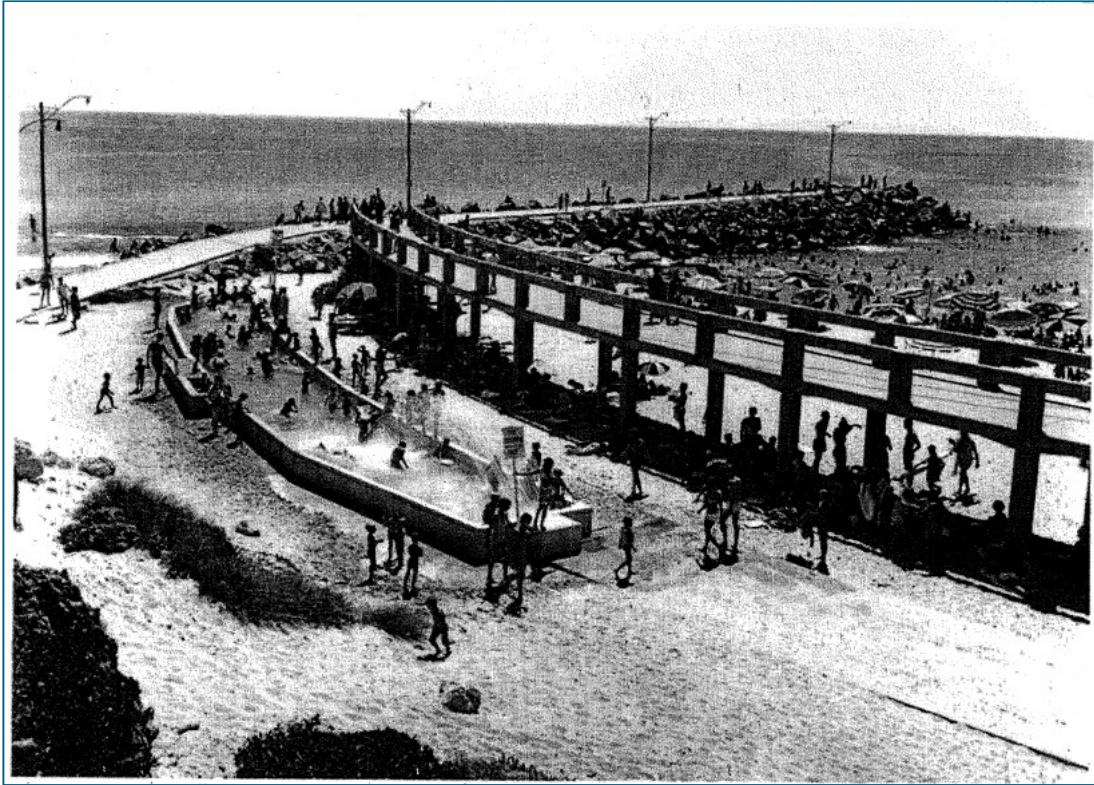
Figure 1-1 Former kids pool located just north of the groyne at Cottesloe
