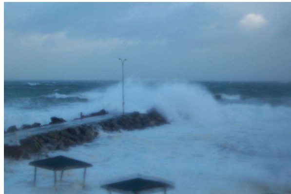
Figure 3-5 Overtopping at the Cottesloe groyne during a winter storm (16 May 2003)
