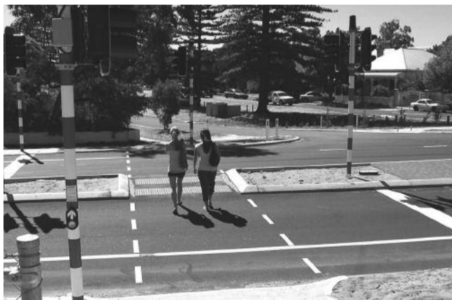
Pedestrian-controlled traffic lights are now fully operational at the Grant Street/ Curtin Avenue intersection, adjacent to the rail station.
