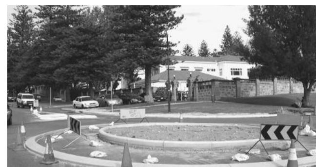
Newly-built roundabout near the Civic Centre aims to improve the Broome Street Black Spot.
