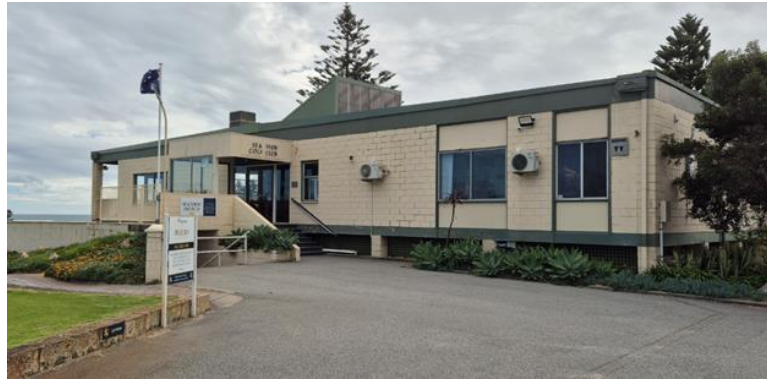
Above: Existing clubhouse (southern elevation)
