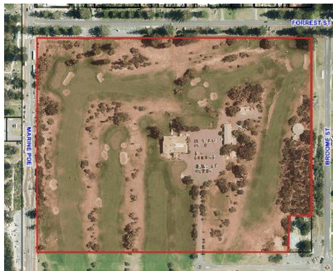
Above: Aerial photo of site
